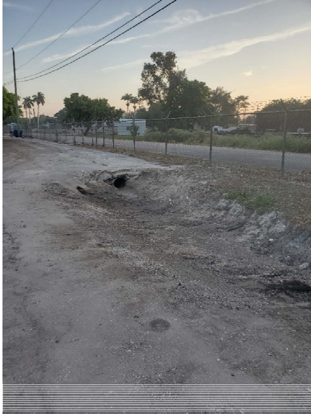
Maintenance yard ditch cleanout.
