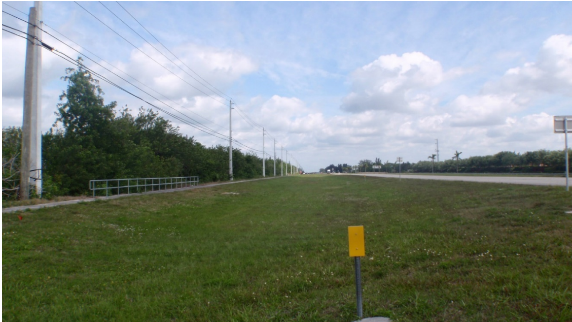
Photo 1: Typical swale on west side of SR 7, northern section of WBID (north of Yamato Road).
