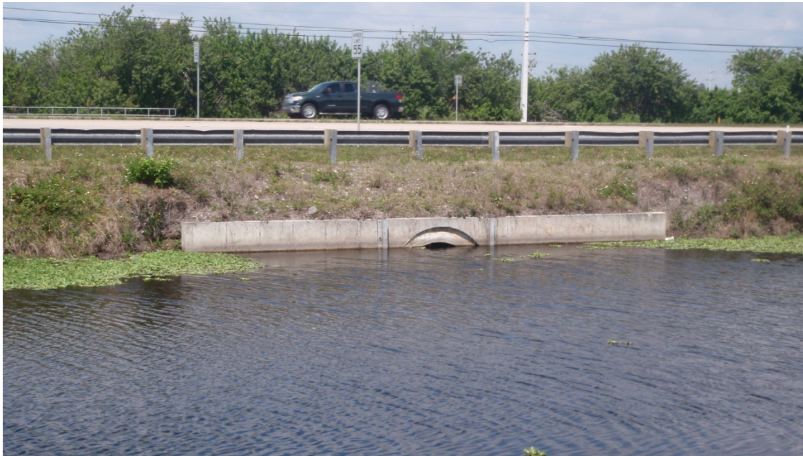
Photo 3: Typical FDOT outfall to E-1 Canal.
