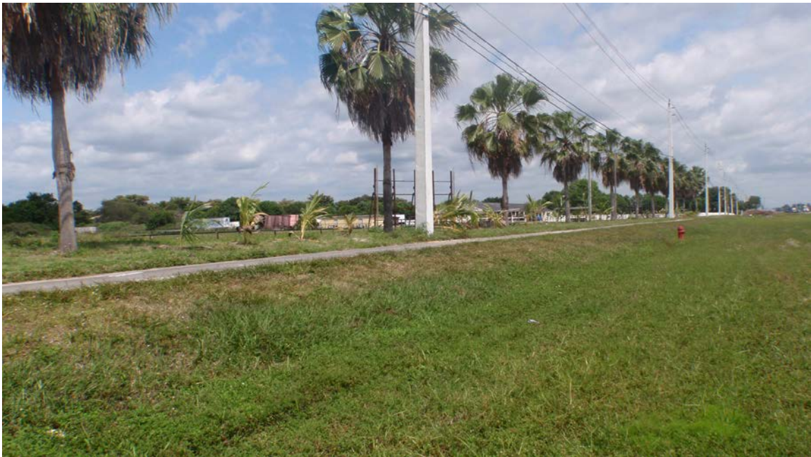
Photo 17: Typical swale in northern portion of WBID on west side of SR 7 between road and agricultural lands. The agricultural lands in this section of WBID drain west, not to the E-1 Canal; however, the swale treats stormwater from SR 7 and drains east to E-1 canal via series of culverts under road (see Photos 2 and 3above.)
