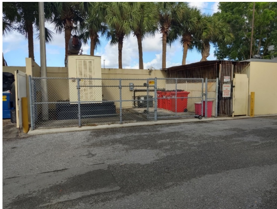
Photo 11: Medical waste dumpsters behind locked gate behind Medical Center.
