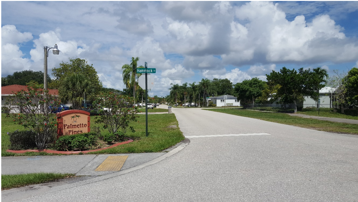
Photo 5: Typical neighborhood on sewer in southeast portion of WBID with stormwater Sheetflow to swales.
