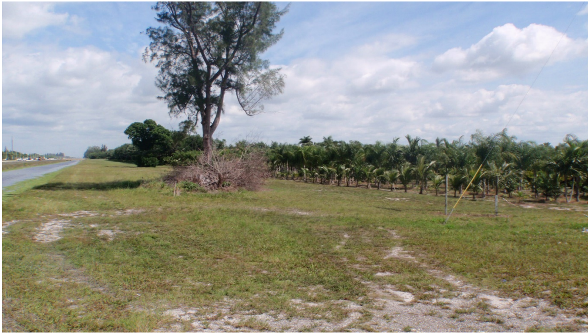
Photo 16: Facing north at SR 806, view of E-1 canal and adjacent tree nursery that drains to east. Typical of well-maintained swale on east side of E-1. SR 7 can be seen in background on far left side of photo, west of the canal. (Note: area east of E-1 canal is actually outside WBID boundary.)
