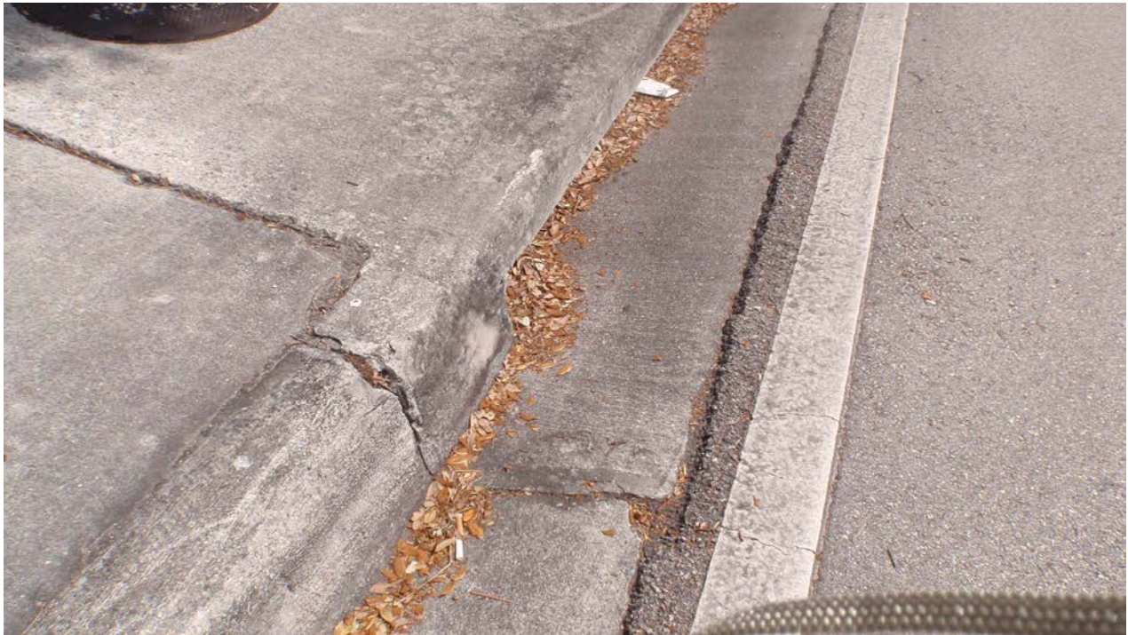
Photo 14: Minor vegetative debris observed along roadways.
