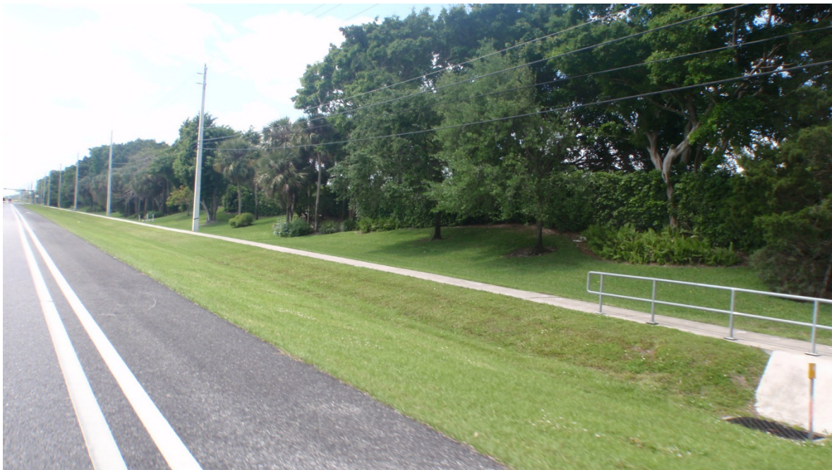
Photo 4: Typical swale on west side of SR 7 in southern section of WBID where west side of SR 7 are primarily single-family home communities separated from SR 7 by landscaped berms.
