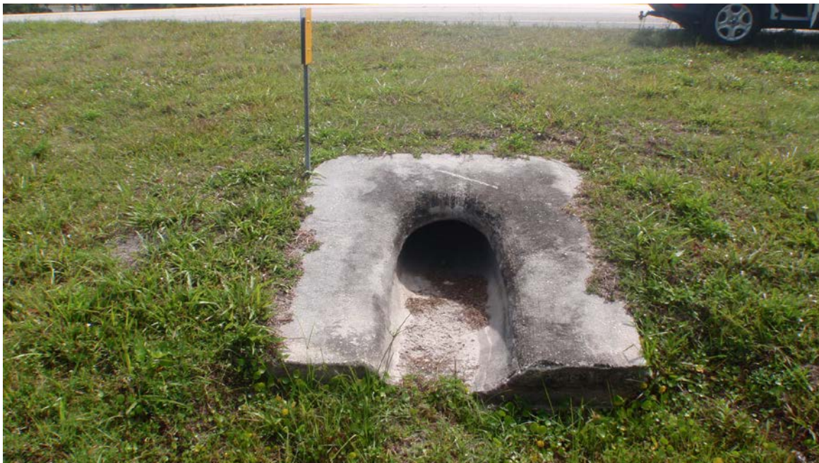
Photo 2: Typical mitered end section in swale on west side of SR 7, connected to culvert that runs east under SR 7 and discharges treated stormwater to the E-1 Canal.
