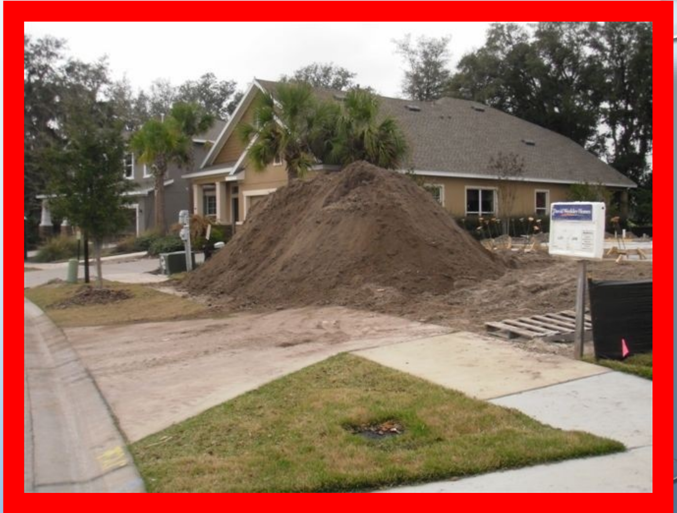
No silt fence or soil stabilization, offsite tracking
