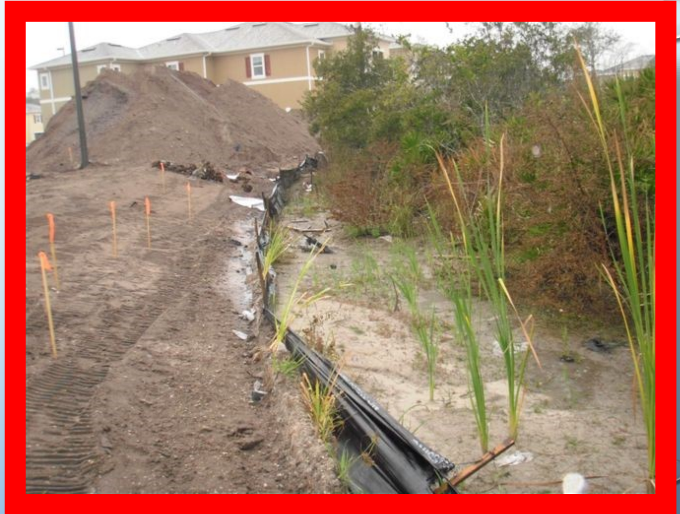
Failing silt fence, no soil stabilization
