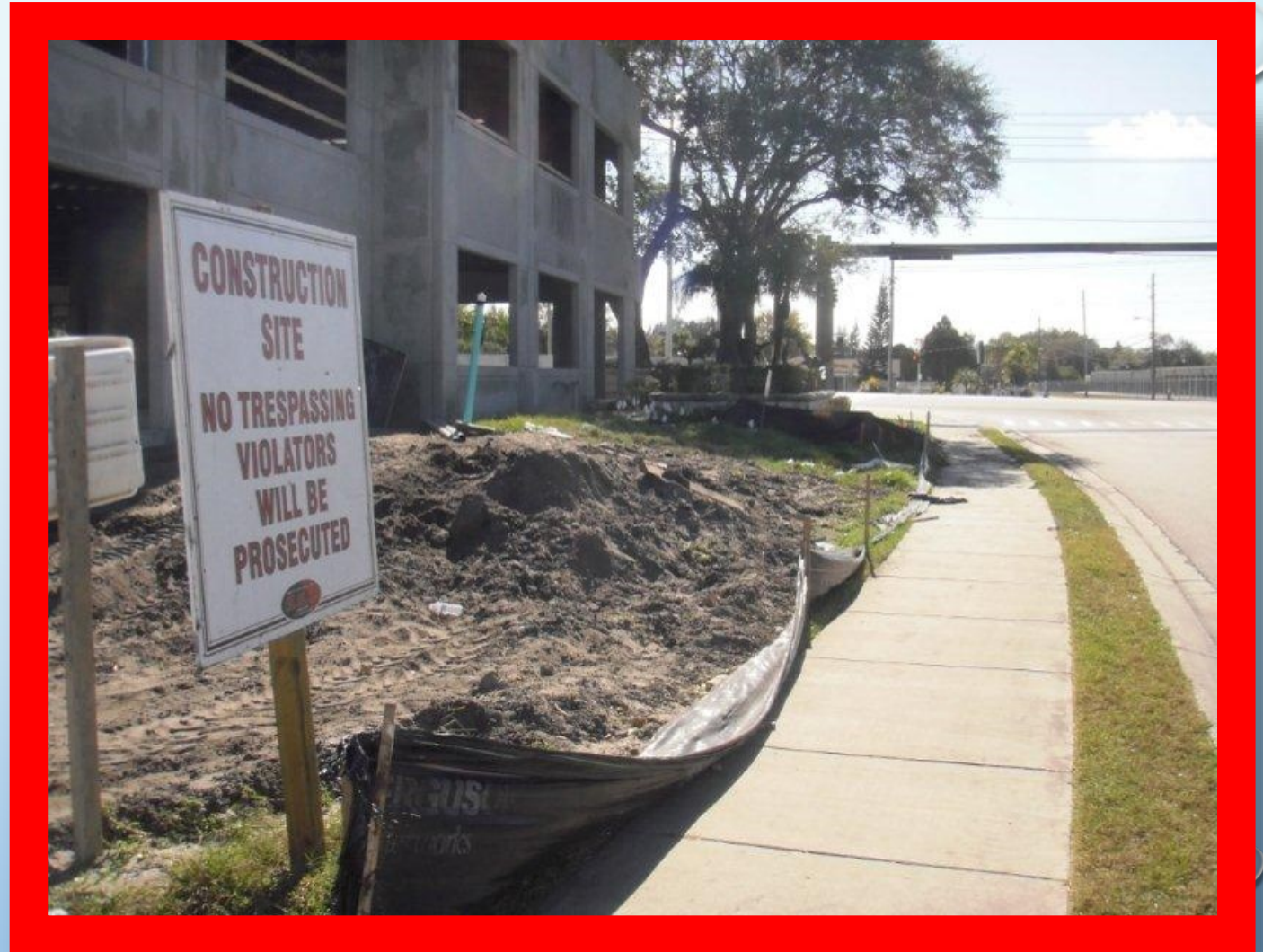
Failing silt fence
