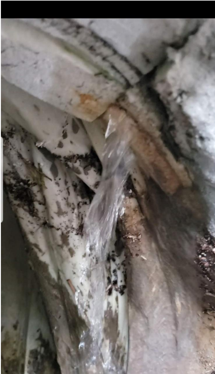
Catch Basin #3 – Leak at 36” Lined Pipe
