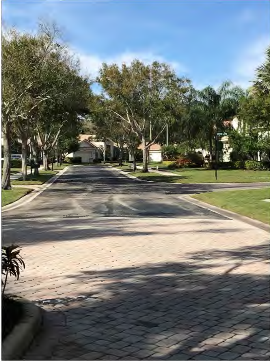
Figure 23. Unit 41 typical roadway with valley gutter system
