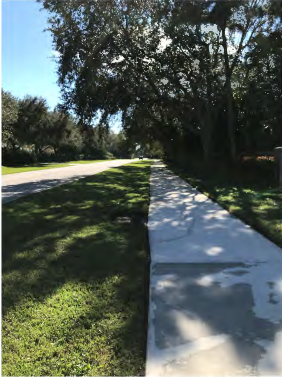
Figure 21. Unit 33 typical grass swale
