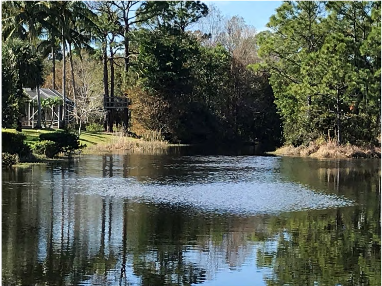
Figure 20. Outfall and Water Quality sample location of Unit 33
