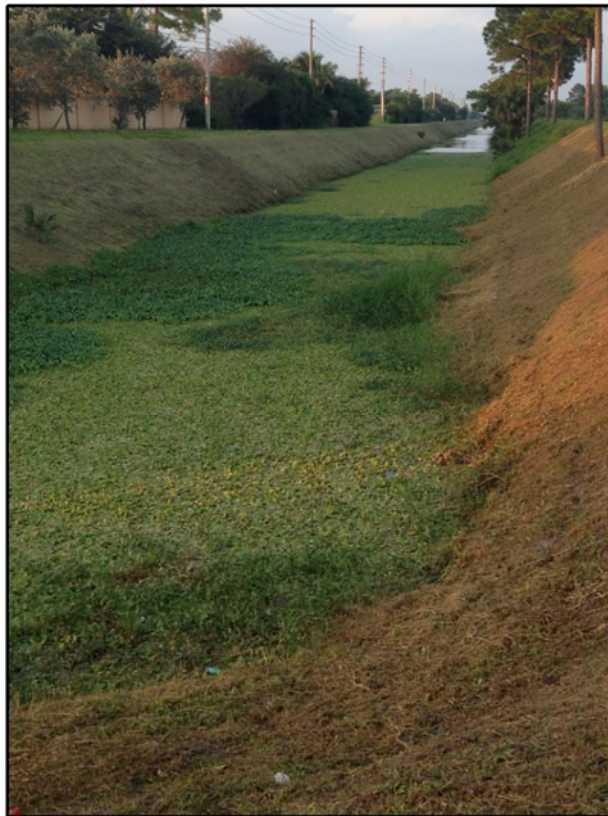
Figure 3-4: Floating Aquatic Vegetation Growth in the North Palm Beach Heights Water Control District (NPBHWCD) Canal (Sims Creek)
