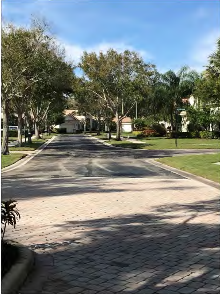
Figure 23. Unit 41 typical roadway with valley gutter system
