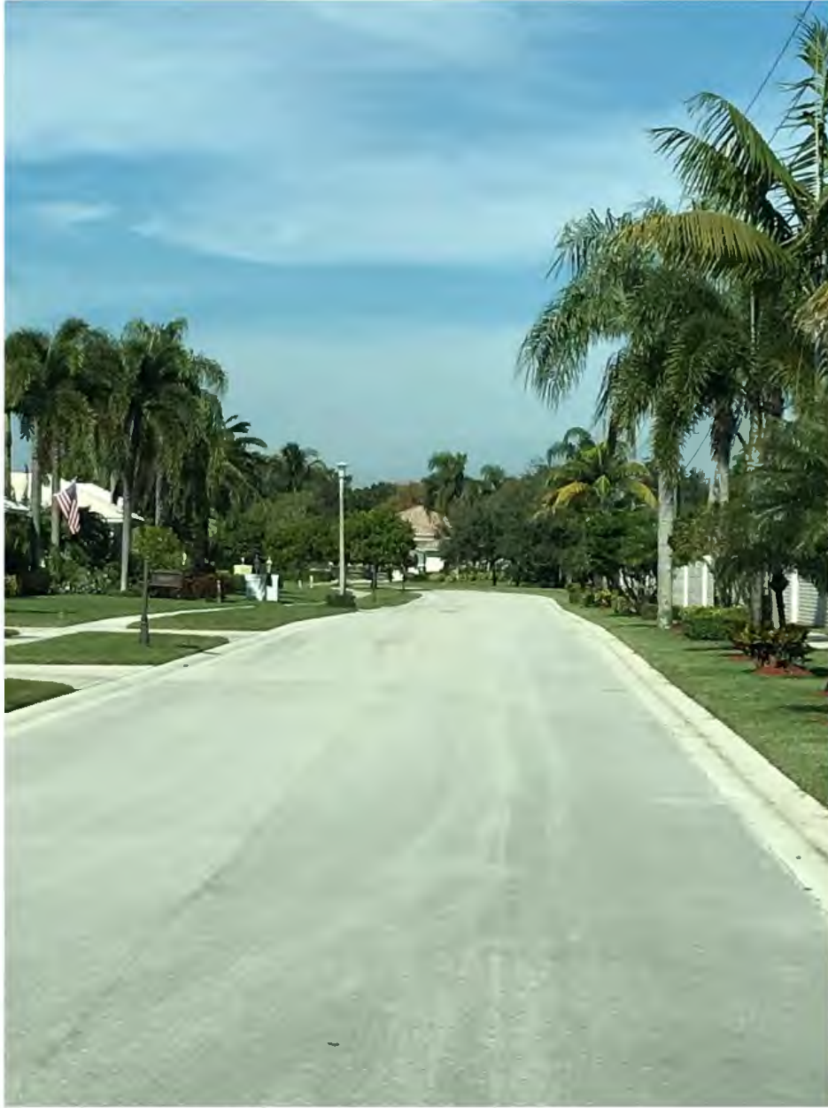
Figure 19. Unit 32 typical road section with valley gutter
